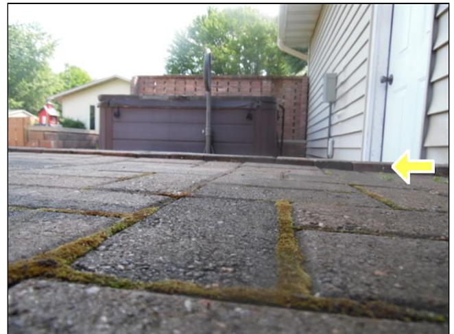
(3) The patio block is uneven at the top step. This is a potential tripping hazard.
