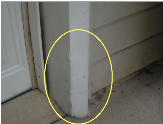
(8) There is loose weatherstripping at the exterior of the overhead door.
