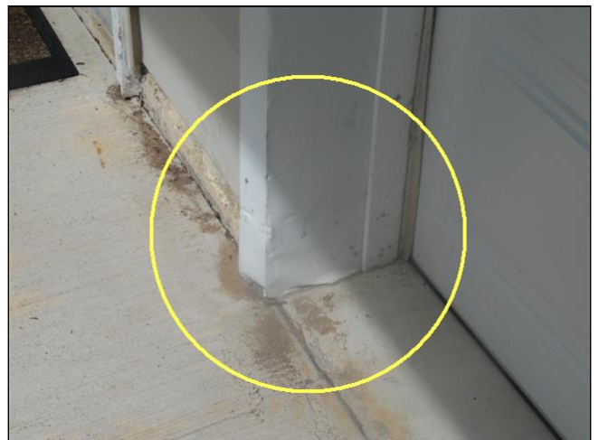
(7) There is impact damage at the bottom of the overhead door jambs and trim.
