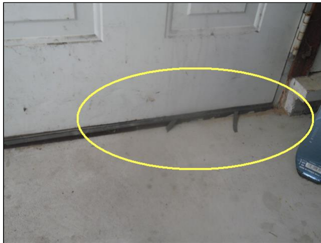
(7) There is impact damage at the bottom of the overhead door jambs and trim.
