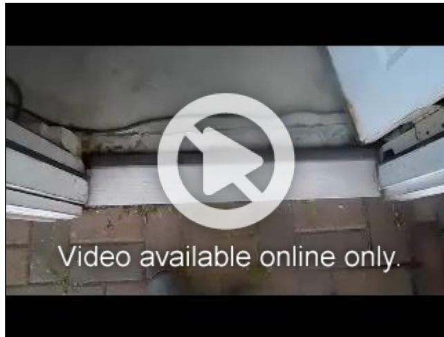
(6) There is damaged weatherstripping at the bottom of the front garage service door.
