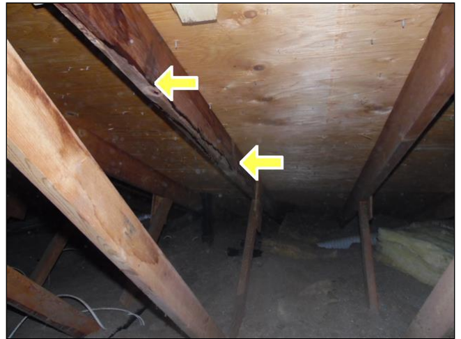
(3) There are old moisture marks in the attic that appear to be where a roof vent once was installed.
