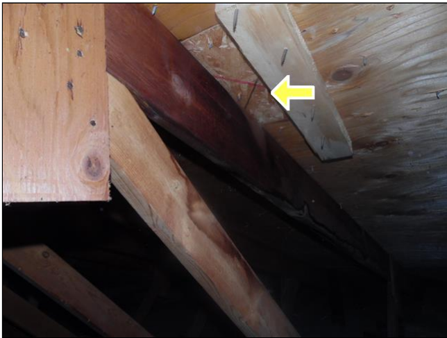
(3) There are old moisture marks in the attic that appear to be where a roof vent once was installed.
