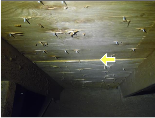
(3) There are old moisture marks in the attic that appear to be where a roof vent once was installed.
