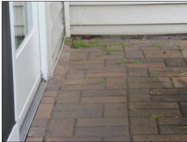
(3) The patio block is uneven at the top step. This is a potential tripping hazard.
